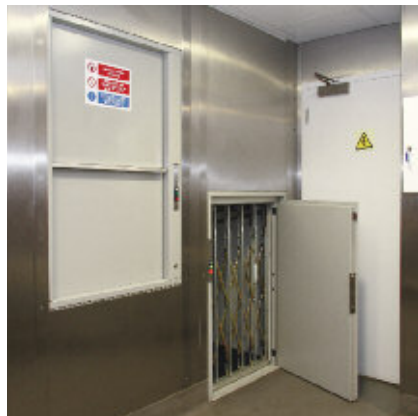
Hinged door option shown on floor serving 100kg model
